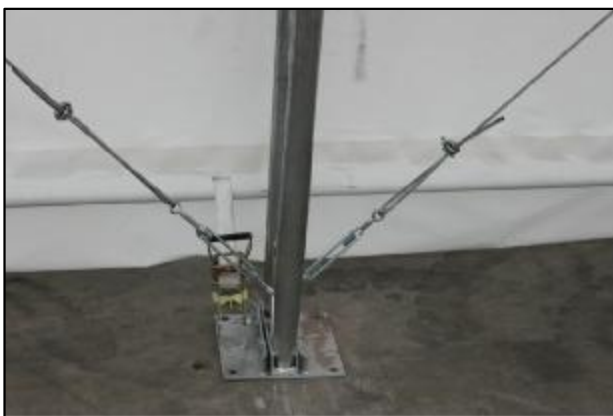
Figure 7 The position of windstabilizers (turnbuckle and cable) at the sidewall.
